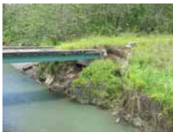
Photo 2.8 Abutment of the Old Ngalimbiu Bridge (1)
