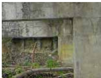
Photo 2.9 Abutment of the Old Ngalimbiu Bridge (2)
