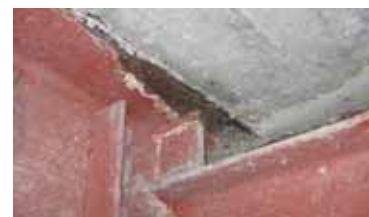
Photo 2.1 Steel elements near bearing
