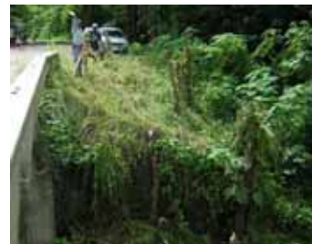
Photo 2.10 Abutment of Tenaru 1 Bridge
