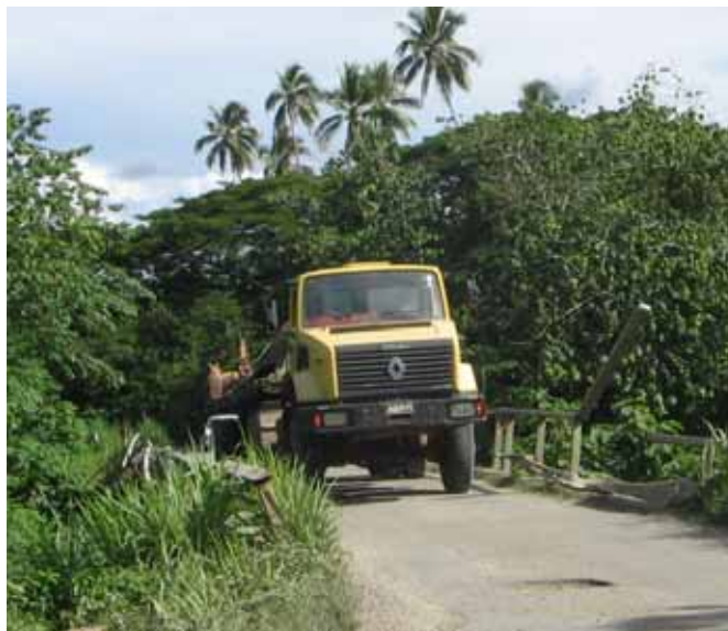
Photo 2.7 Heavy trailer passing Tenaru 2 Bridge
