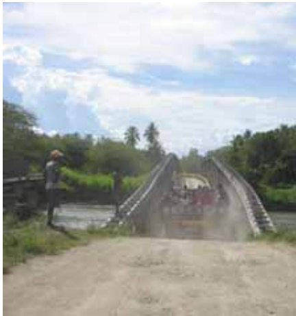
Photo 2.4 Truck passing the existing Ngalimbiu Bridge
