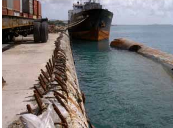
Photo-2.2-1 Existing Condition of B Dock Superstructure
