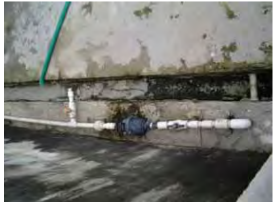
Exposed water meter. Service pipe is exposed and there is no cover of meter.
