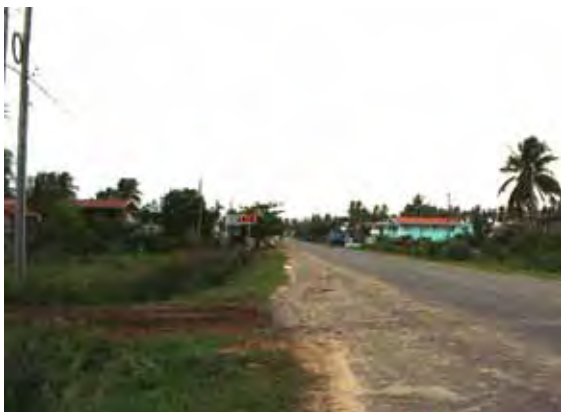
Suburb area of the Project area. The existing distribution trunks run along both road shoulders.
