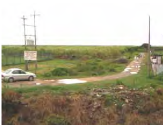
Site for Queenstown WTP. Presently sugar cane field surrounded by ditches. Access road will be construct by infilling the ditch. No house around.
