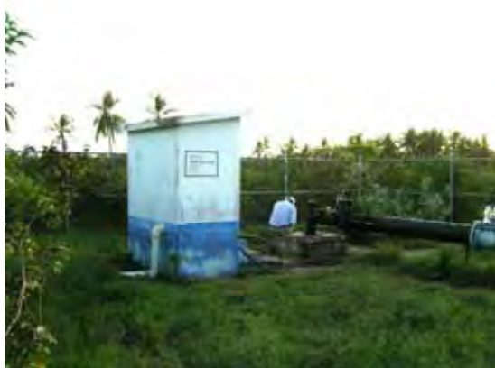
Existing No.57Village pumping station. This well is a water source of the No.56 Village WTP.
