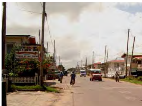
Close set area in the Project area. The existing distribution trunks run along both road shoulders.
