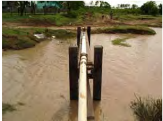
River crossing by wooden pile. Locally available hard wooden pile is resistant to corrosion. River crossing by wooden pile is common works in GWI.
