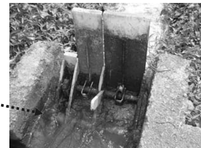
2. Water level measurement bar - How to check water level
