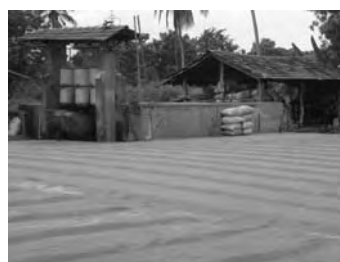
Medium Scale Commercial Rice Mill (Parboiling facility and paddy sun drying yard)
