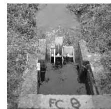
Gate of 10L is open at the turn-out of FC-8.
