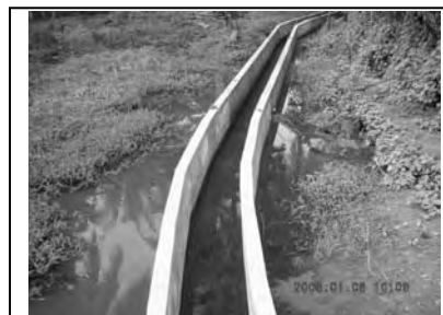
Left Bank Main Canal Recently Rehabilitated under NWS&DB (Thuruwila Medium Scheme)
