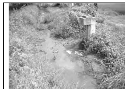
D-Canal 1 in LB Tract 2 Sedimentation and Vegetation inside (Rajangana Major Scheme)
