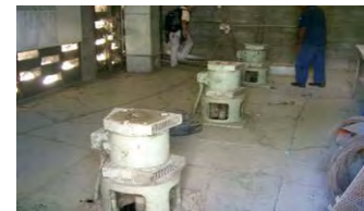
Point Cruz Pumping Station
