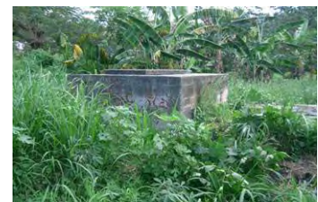
Vara Creek Communal Septic Tank
