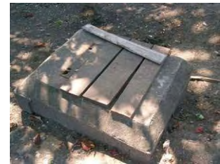
Naha Valley Manhole
