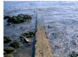
Mbua Valley Outfall
