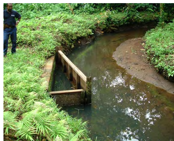
Situation of water-intake of Ziata river. The river has enough discharge to meet water demand of 2010. There is an existing purification plant 200m north of this intake.
