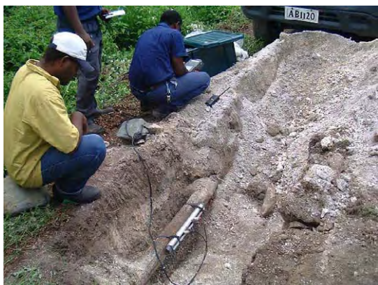
Situation of leakage measurement work before pipe replacement at Kukum Campus.
