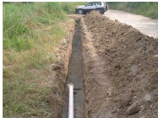
Situation of pipe replacement work at Kukum Campus.
