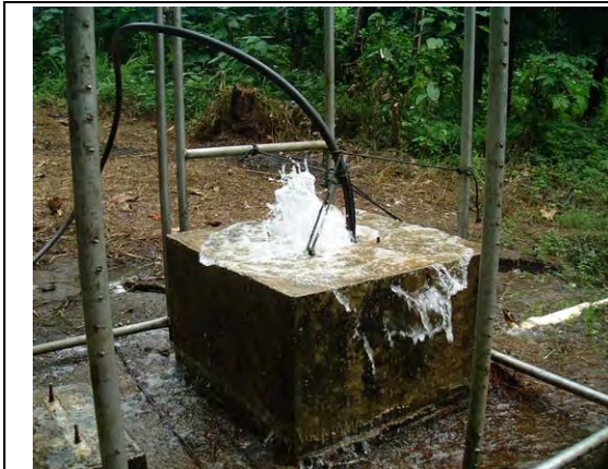
Situation of borehole washing in White river area. Several boreholes were washed to recover production capacity in the Study.
