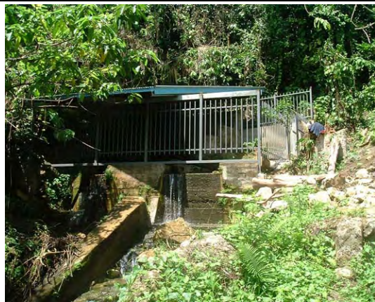
Situation of Konglai Spring in Dec. 2007. Discharge rate from the spring has been reduced since Nov. 2006 as half as the normal condition. Almost all the water is being taken by SIWA results in little over-flow.
