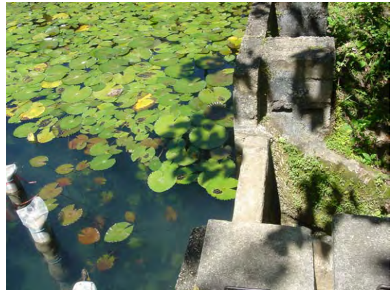
Condition of water intake point and weir of Rove Spring. Water weed can be seen and water quality is acceptable.
