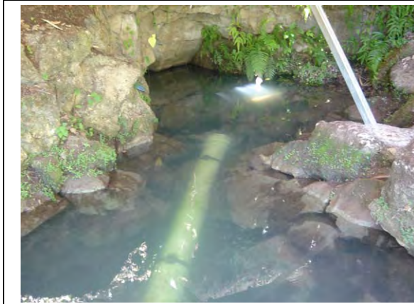
Water intake point of Konglai Spring. This spring is the main water source for Honiara covering 50% of distribution volume. However, the distribution volume is reduced to less than 40% due to the blockage occurred in October 2005.
