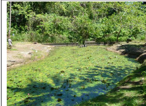
Rove Spring which is one of three springs in Honiara. Intake volume of this spring is as small as one-seventh of Konglai Spring. Water from the spring is distributed mainly to Point Cruz district.
