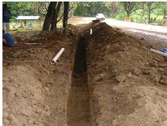
Situation of pipe replacement work at Kola Ridge.
