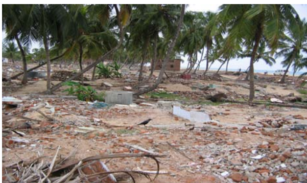
Kalmunai - Tsunami Destruction of Coastal Housing
