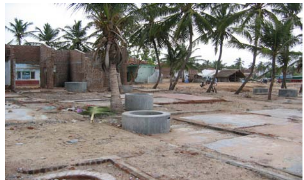
Kalmunai - Tsunami Destruction of Coastal Housing
