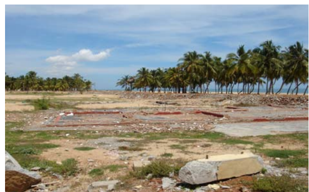
Kalmunai - Tsunami Destruction of Coastal Housing
