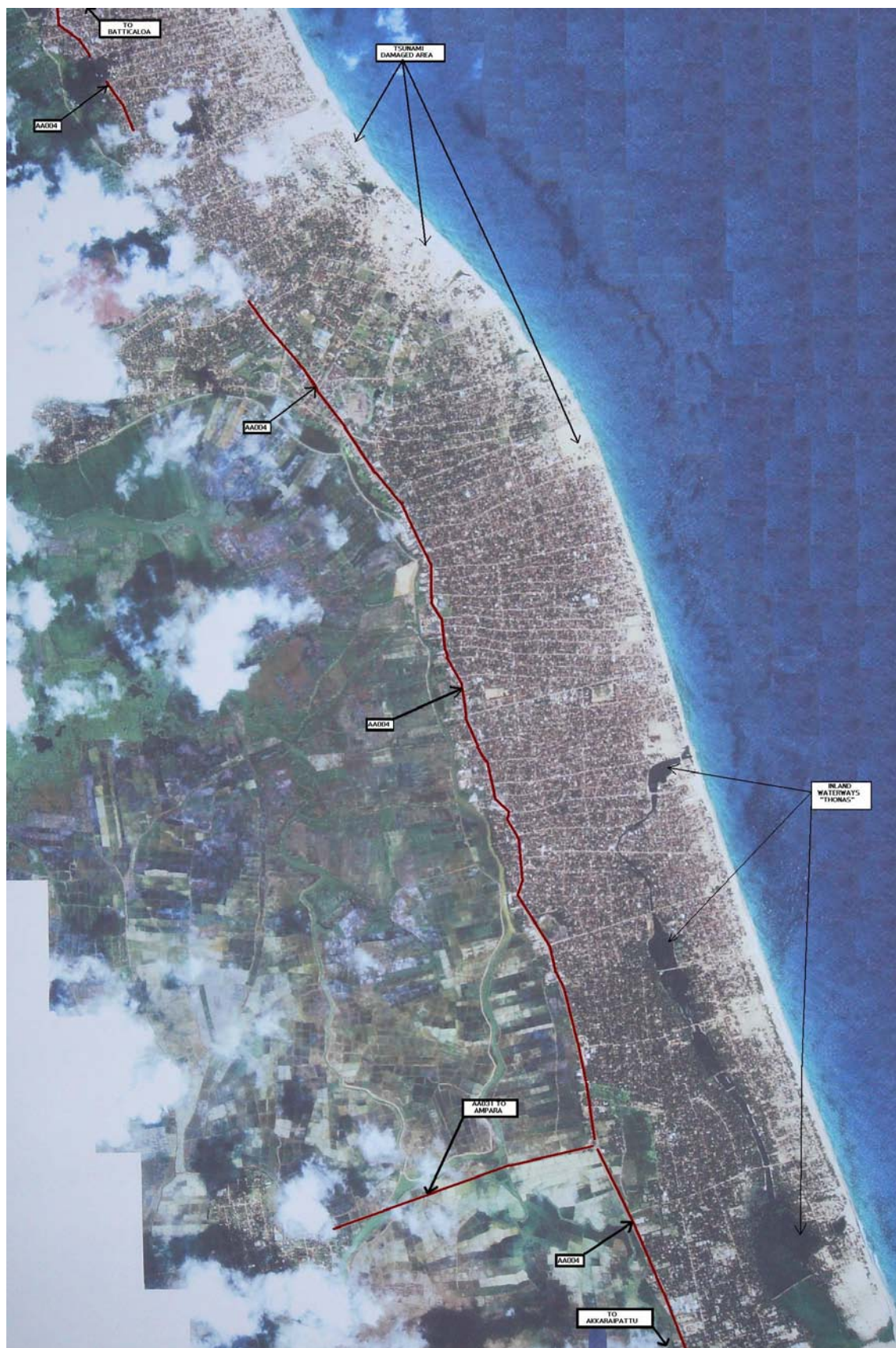
Figure 16.2.1. Aerial Photo of Post-tsunami Kalmunai Township
