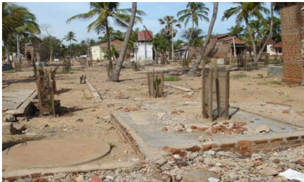
Kalmunai - Tsunami Destruction of Coastal Housing
