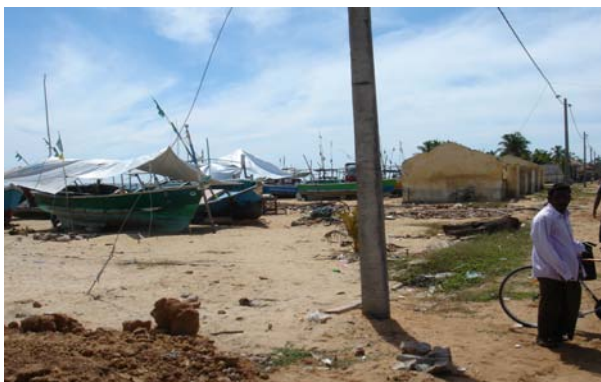
Kalmunai - Tsunami Destruction of Coastal Housing
