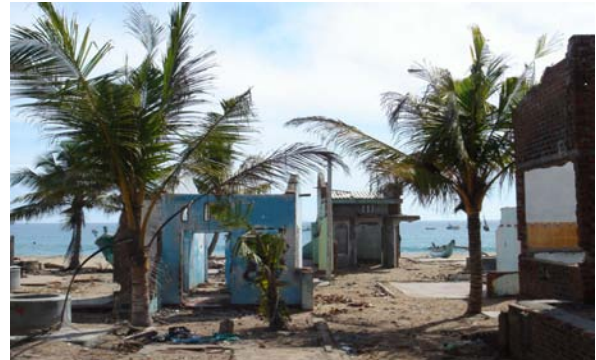
Kalmunai - Tsunami Destruction of Coastal Housing
