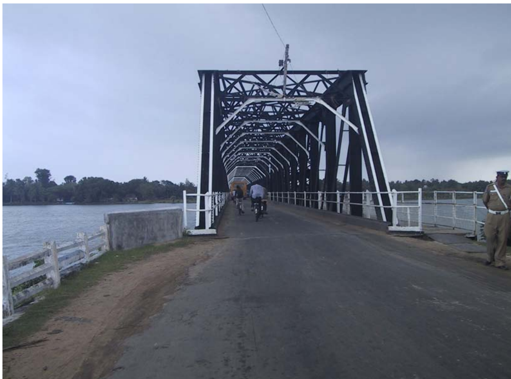
Figure 8.4.1. Existing Kallady Bridge from North Embankment
