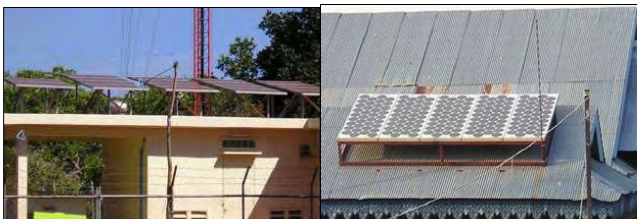
(a) Medium scale PV system at telecom center (b) Small scale PV system at repeater station
