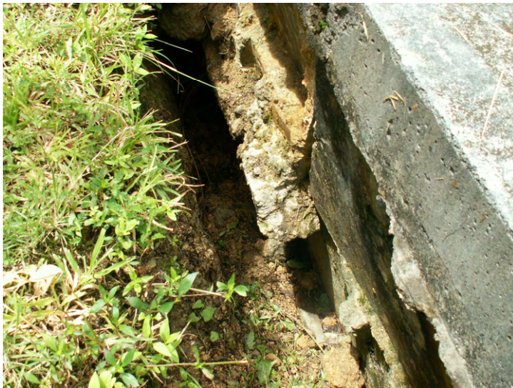
Some parts of the channel were completely isolated from the soil (Photo 2)
