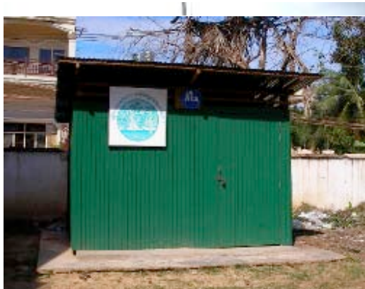
Store house built at Hun Sen Primary School
