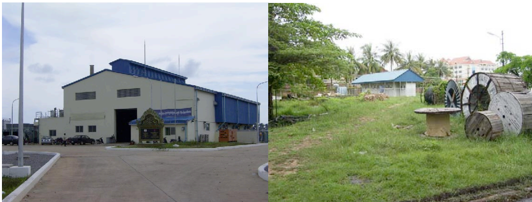
Existing Power Station (new)
