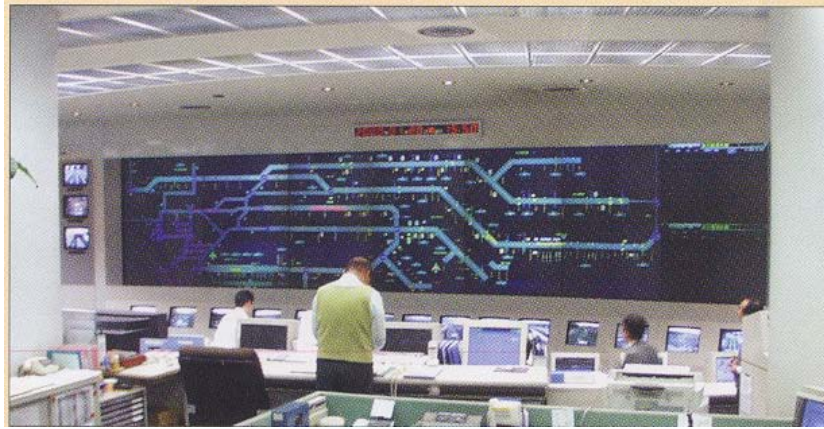
Figure 8.3-2 Example of Traffic Control Center in Japan
