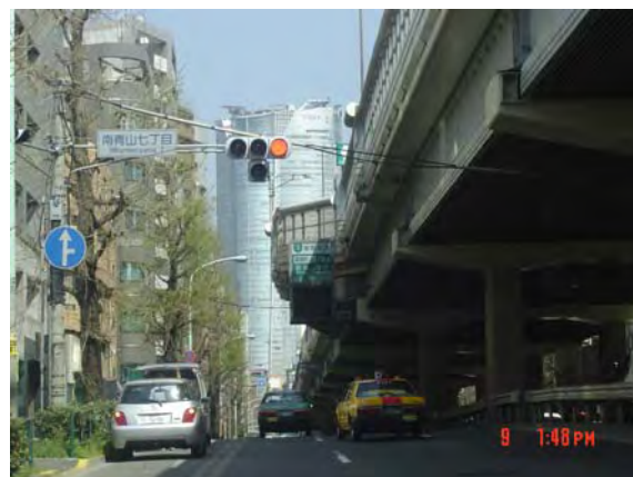
Emergency Telephone Space Tokyo Metropolitan Expressway
