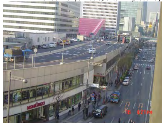
Shopping Centre Under Tokyo Metropolitan Expressway
