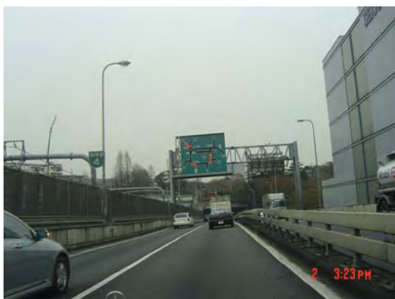
Guiding Changeable Sign Tokyo Metropolitan Expressway
