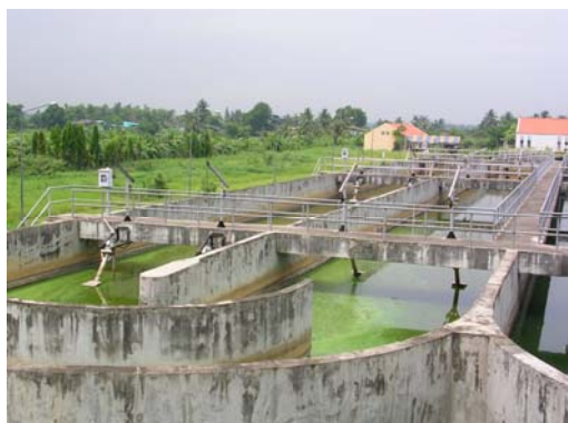
5. Pathumthani STP (Oxidation Ditch) (Before rehabilitation)
