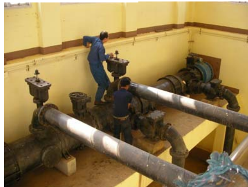
2. Inspection of check valve conditions
