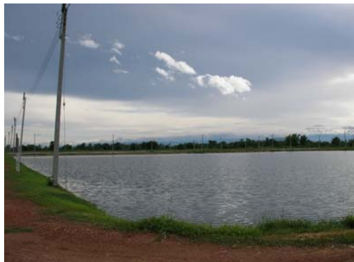
1. Kampaengphet STP (Stabilization Pond)
