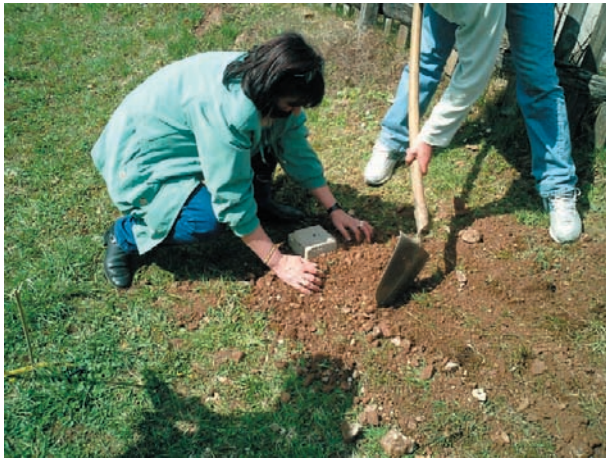
Photo 2 - 5 New Control Point Establishment 1
