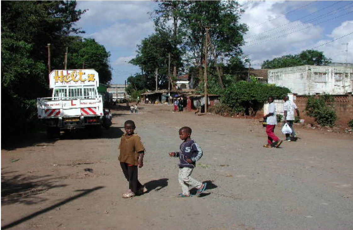
Missing Link No.4: At the northern end of Mpaka Road, a few kiosks occupy the road reserve.
