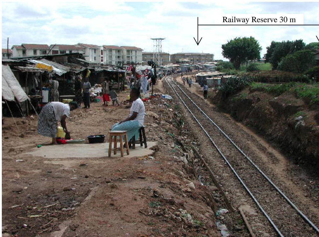
Missing Link No.15: Encroachment of the local residents into the railway reserve near Mbagathi Way.
