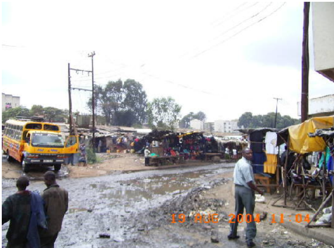
Missing Link No.1: At mid point, road reserve is heavily occupied.
