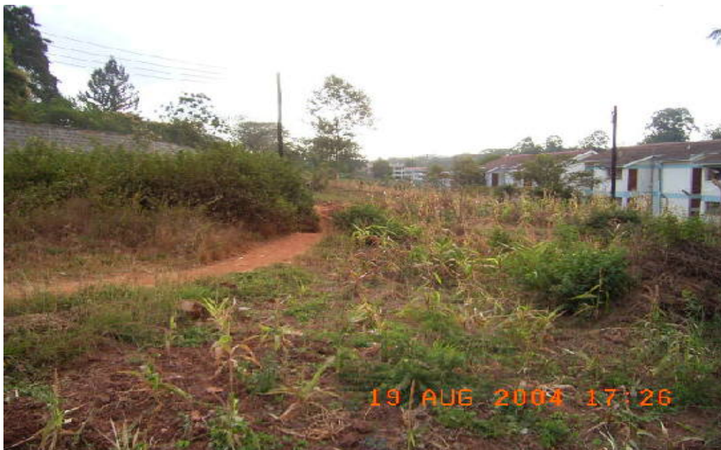
Missing Link No.15: No occupation of the road reserve at mid point.
