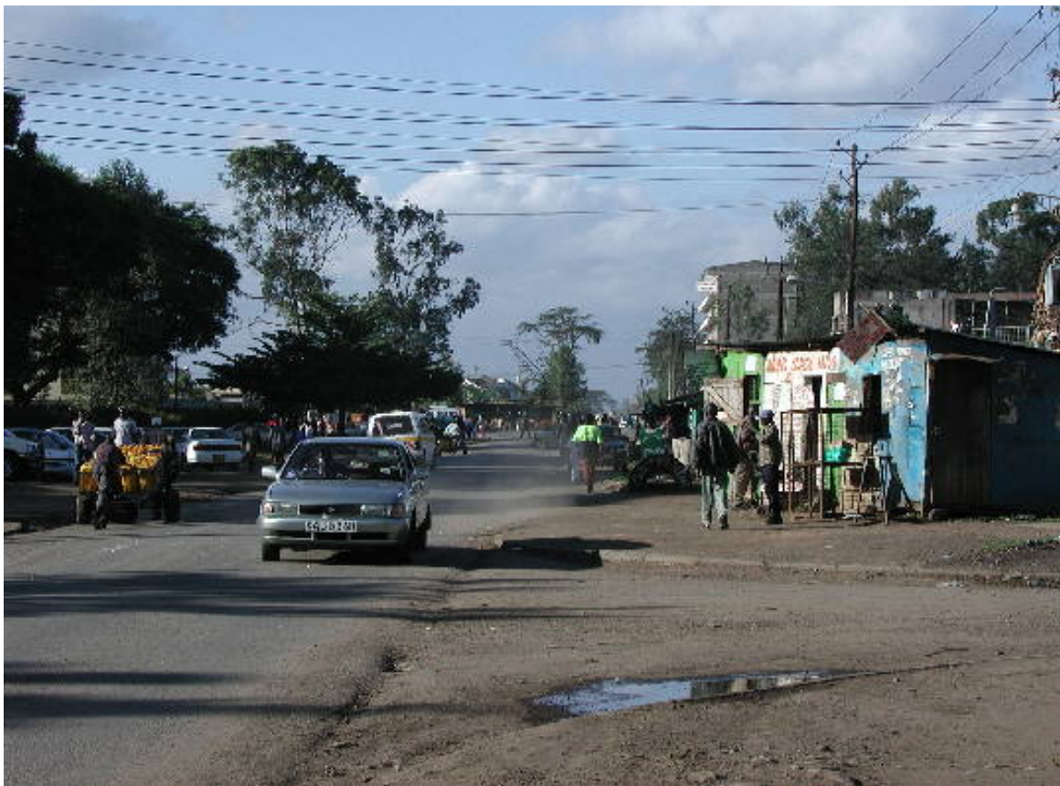
Mission Link No.5: From north to south, large part of the road reserve is occupied by kiosks.
