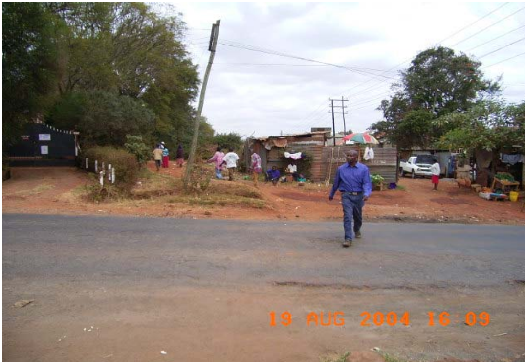
Missing Link No.7: A few temporary structures occupy at this section of Gatundu Road.
