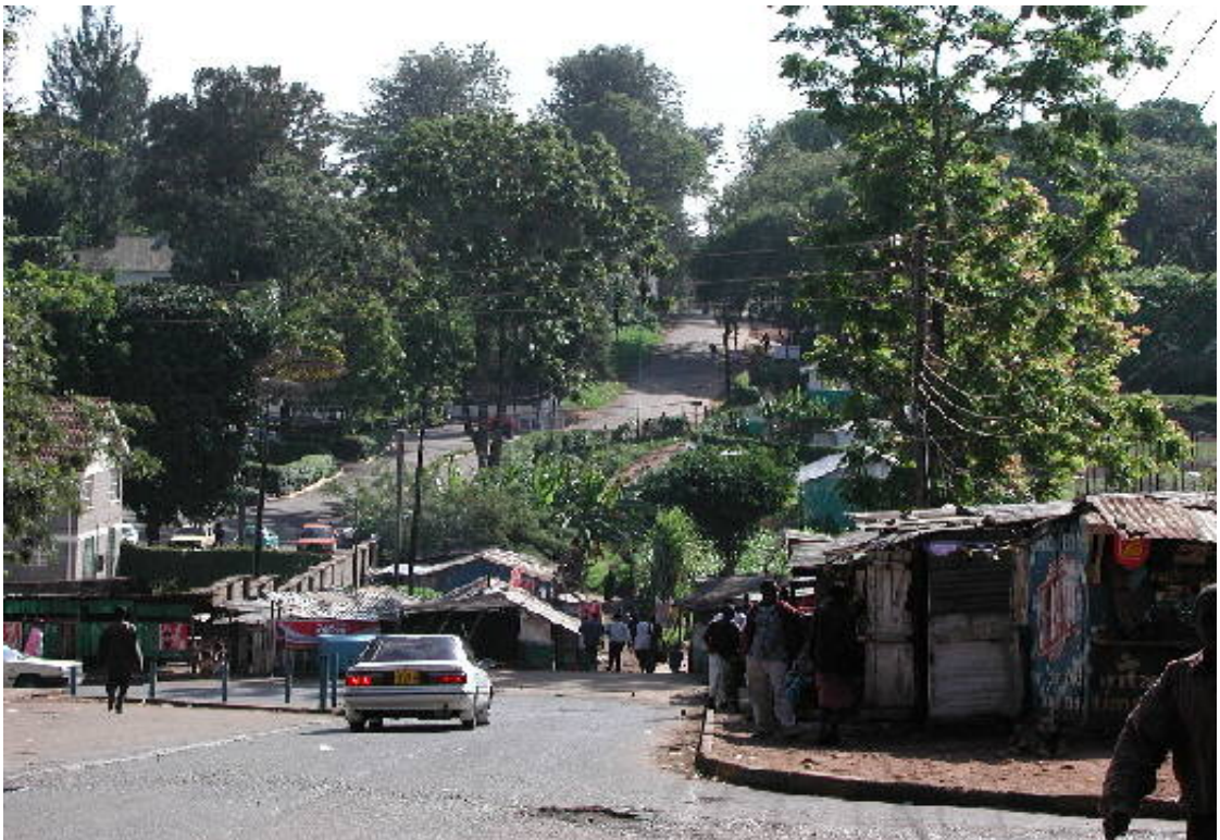
Missing Link No.4: At the southern end of Mpaka Road, a school occupy the road reserve. Outside the school kiosks also occupy the road.
