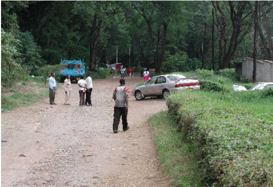
Missing Link No.9: At Denis Prit Road, gardening occupy the road reserve.
