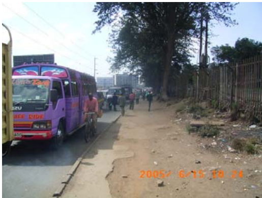
NMT: No pavement. State of Negligence
