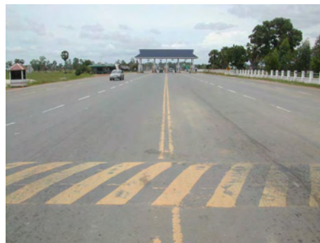
A. Front View of Toll Gate
