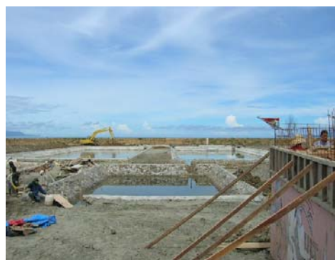
Overview of rehabilitation works on Septage Treatment Plant
