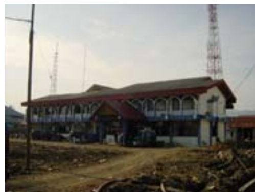
Figure 1.1.2 Appearance of the RRI Studio after the Disaster
