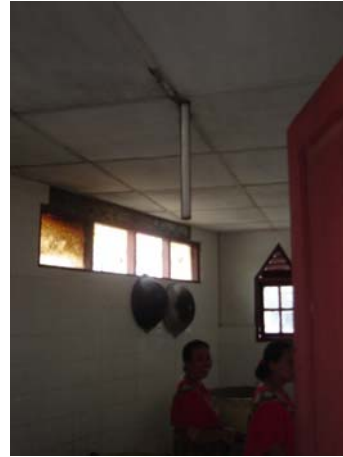
Lighting fixtures in sleeping rooms and kitchen (the screws holding the fixtures in place have dropped out and the fixtures are hanging by their cables)
