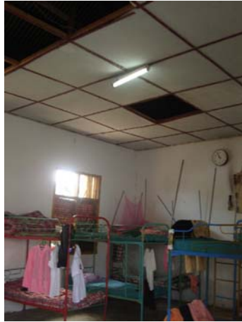
Lighting fixtures in sleeping rooms and kitchen (the screws holding the fixtures in place have dropped out and the fixtures are hanging by their cables)
