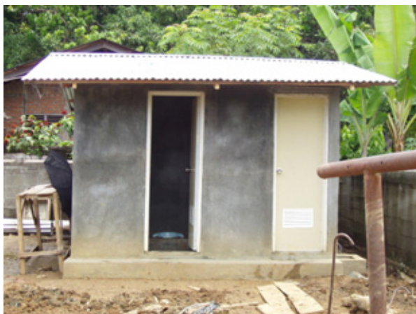
Project No.3 YDD: Sanitation Facility
