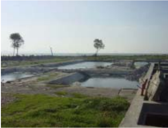
Damaged Human Septage Treatment Plant
