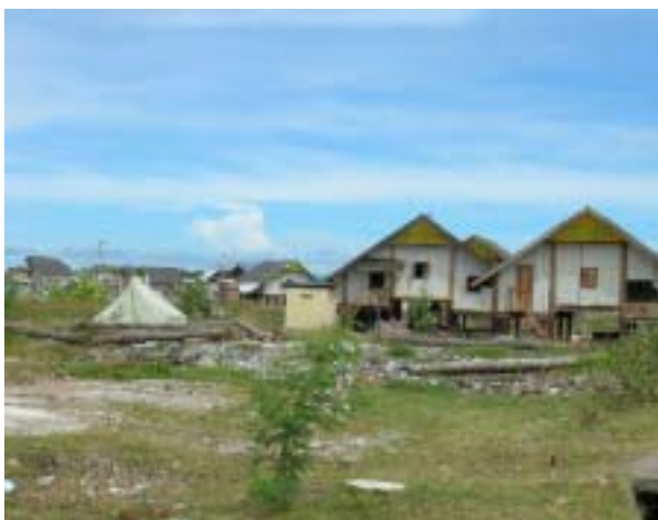
Construction of Permanent Houses
