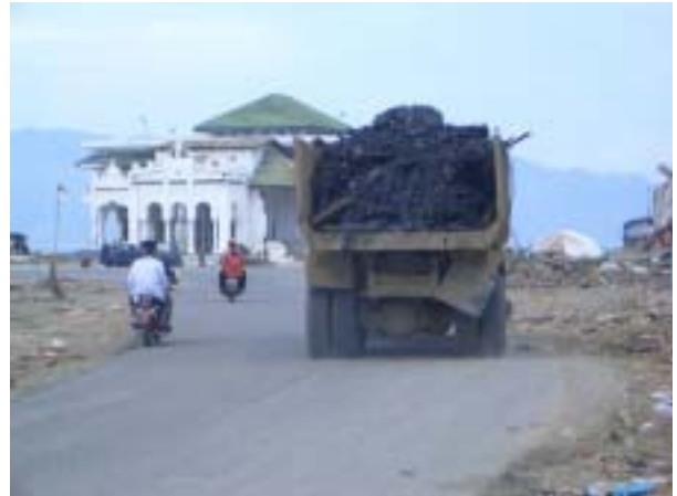
Cleaning of Debris
