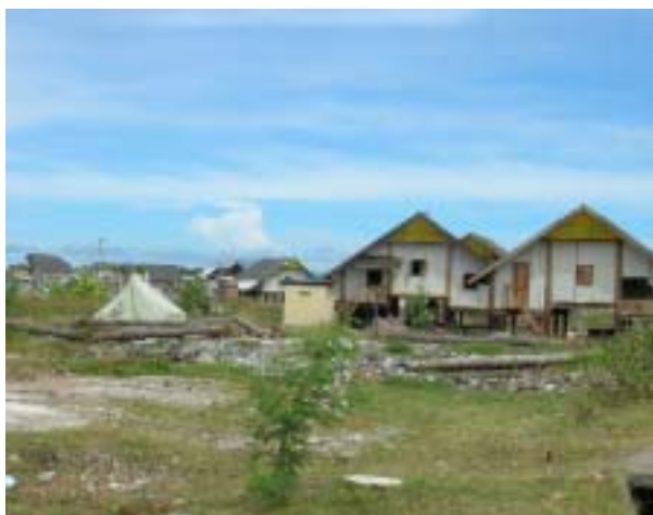
Construction of Permanent Houses
