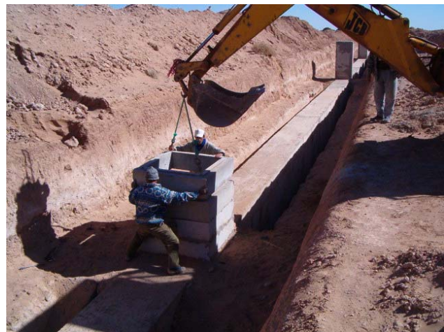
Prefabricate concrete used at khattara Oustania
