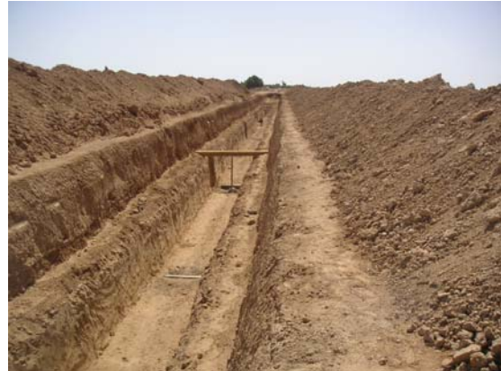
Excavation works along the gallery
