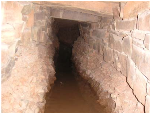
Galley section before rehabilitation works. Riverbed deposits caused leakage before construction.
