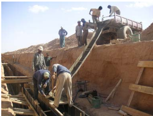
Concrete placing with chute
