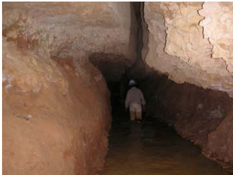
Inside of gallery after widening
