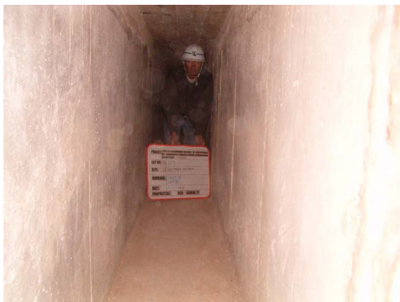
Inside of concrete culvert Width: 0.6m, height: 1.5m
