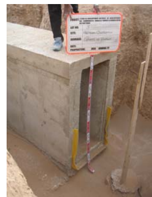
Gallery and vertical shafts of interval 30 m ( Downstream portion )
