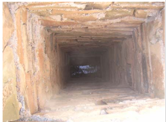
Inside of vertical shaft Shaft has its depth of 5.85m.
