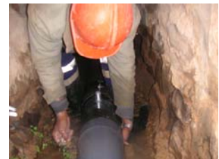
Installation of air pipe
