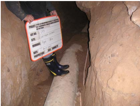
PVC pipe installed along the gallery
