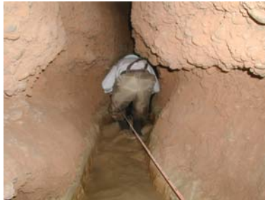
Gallery before rehabilitation work
