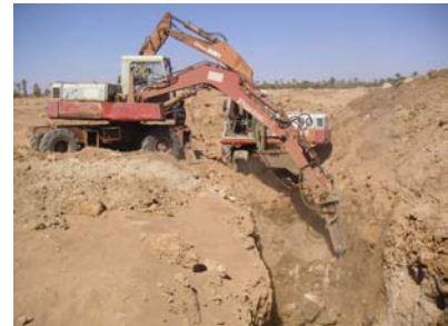
Excavation by backhoe and giant beaker for rock excavation
