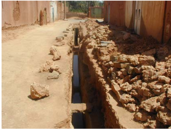
After excavation along the gallery
