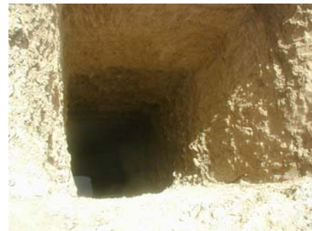
↓ Excavation for masonry protection
