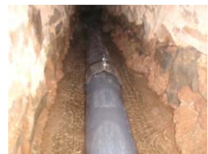
PVC pipe installed in the gallery (diameter 200mm)
