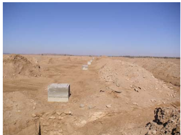
View of ground surface after refilling
