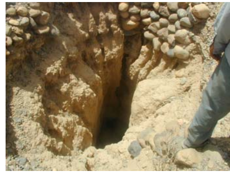
↓ Vertical shaft damaged by floods
