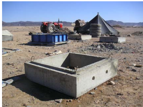
Pre-fabricated concrete for the shaft of khattara
