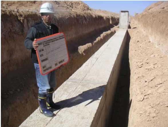
Gallery and vertical shaft with its interval of 30 m
