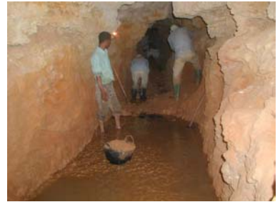
Excavation works in the gallery
