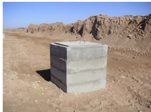
Installation of pre-fabricated concrete
