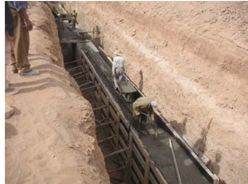
Concrete placing of top slab
