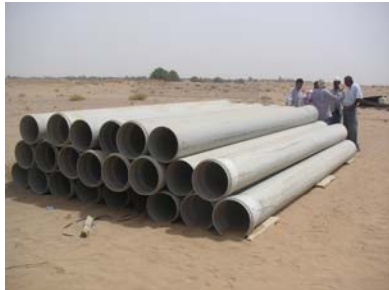
PVC pipe (diameter 400mm) mitigates leakage loss through gravel layer.
