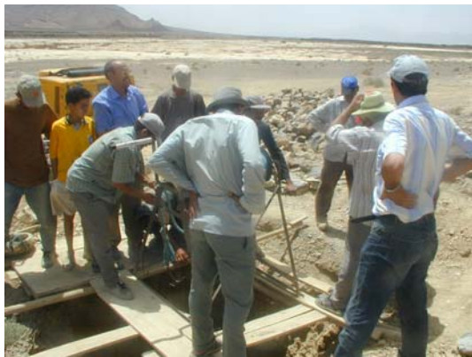
View of rehabilitation works
