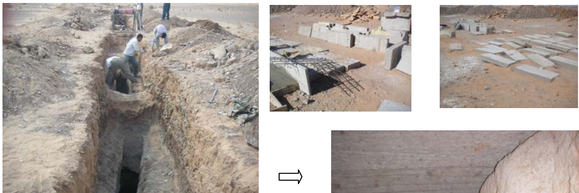
Space between side wall and rock is filled with concrete.
