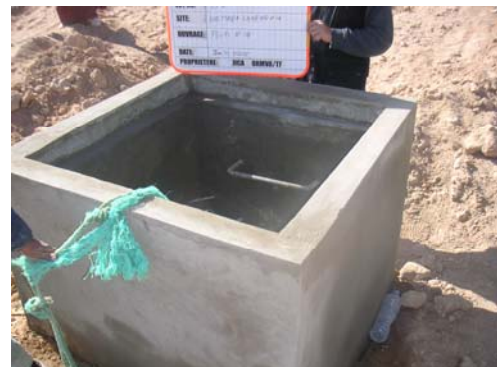
Top of vertical shafts (0.9 m x 0.9 m inside)
