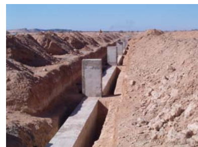
Gallery and vertical shafts of interval 30 m ( Downstream portion )
