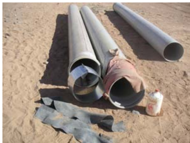
Openings are installed to remove sediments inside of the pipe.
