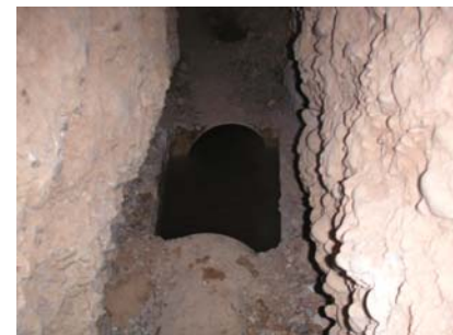
Openings are installed to remove sediments inside of the pipe.
