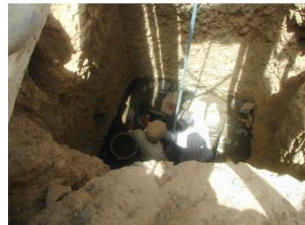
↓ Placing masonry protection in the shaft
