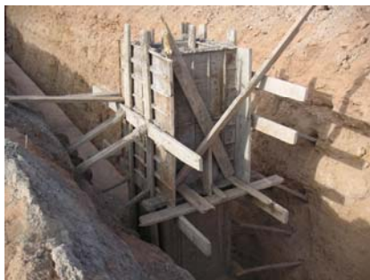
Form assembly for the vertical shafts
