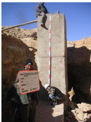
Vertical shaft about 5 m high from the foundation
