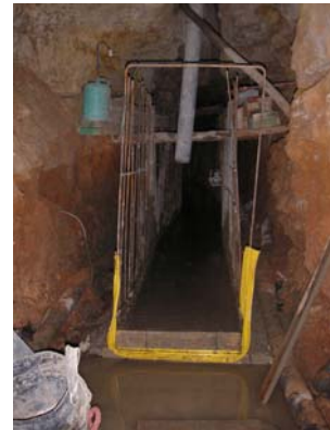
Installation of reinforcing bar and water stop
