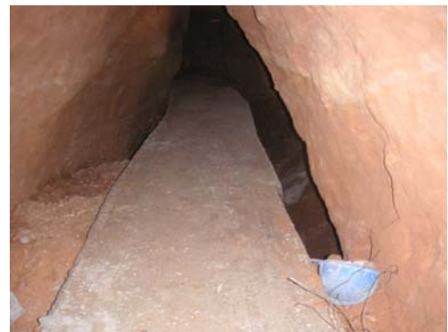
Top surface of concrete culvert
