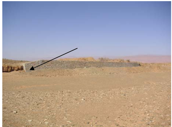
Masonry wall for flood protection (50m length) Gallery is located along arrow mark in the photograph.
