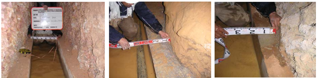
Space between side wall and rock is filled with concrete.
