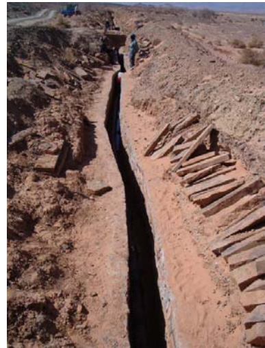
After rehabilitation works by masonry. (same location as photograph at left)
