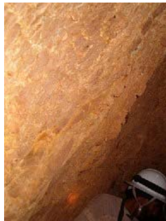
Condition of the downstream Weathered Argillaceous Schist (Vertical bedding)
