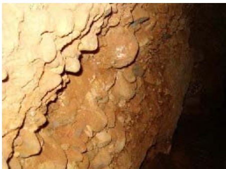
Calcareous cemented gravel and boulder formation in the upstream (seepage formation)
