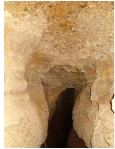
Condition of the khattara upstream Gravelly portion and sand portion layer horizontally
