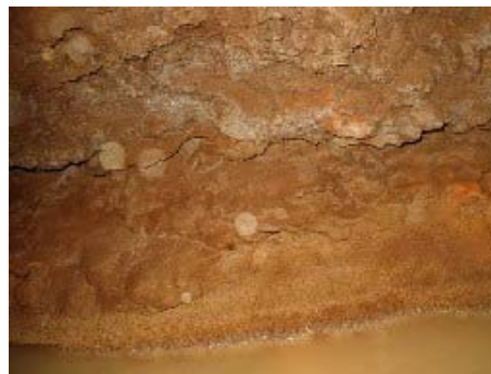
Condition of cementation by limy material just above water seepage level.
