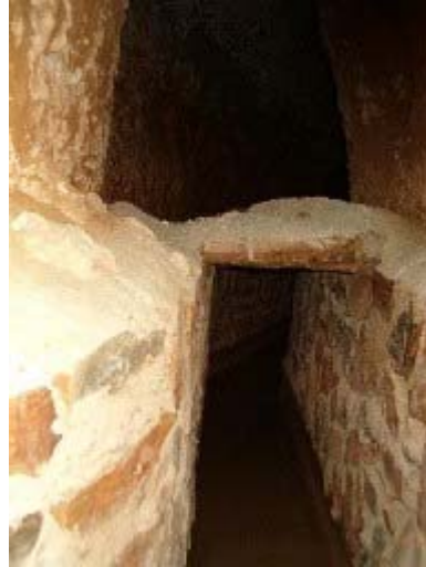
Khattara downstream is protected its sidewall by masonry and platy rock ceilings preventing for deposits in the bottom of falling soils from top wall.
