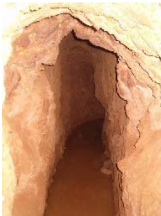
Condition of the downstream Lithological condition around khettra is very different from the up- and midstream. It dug through completely in bedrock, then very stable
