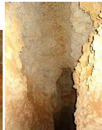
Condition of cementation of calcareous gravel (top wall)
