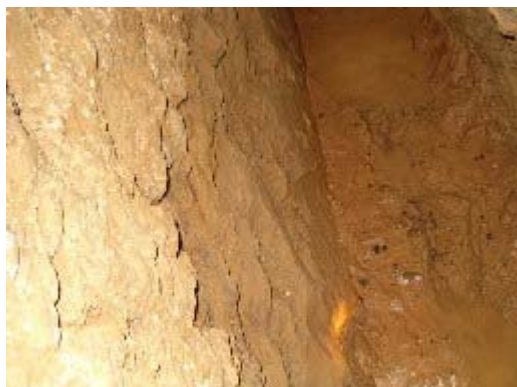
Condition around the Mother Well. Bedrock of the bottom and side wall and gravel layer of upper side wall portion. Very few water.
