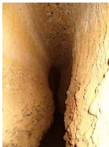
Condition of gravel and sand layers in the upstream portion
