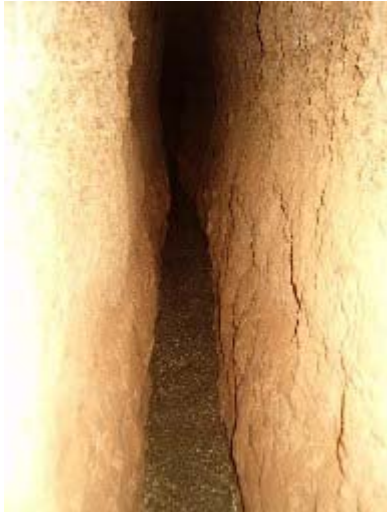
Condition of khattara downstream (Clayey soil)
