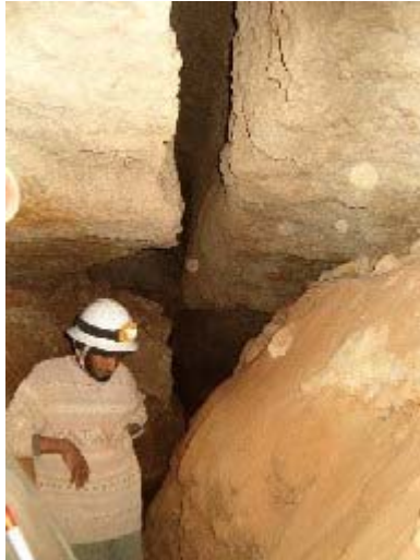
The upper is cemented layers and the lower is brittle sand (downstream)
