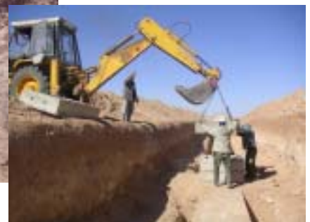
Vertical shaft work using pre-fabricated concrete
