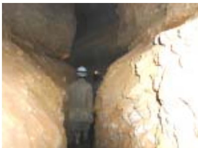
Galley before rehabilitation (Gallery wall is susceptible to collapse)
