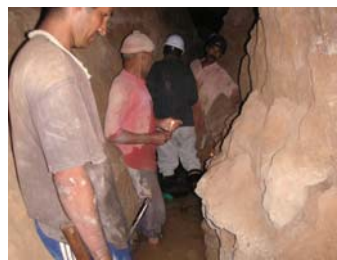
Rehabilitation of khettara (Tunnel works)
