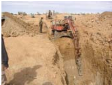
Open excavation works by excavator and rock beaker
