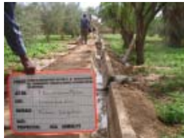
Canal rehabilitation work by concrete lining canal About 10% increase of irrigation efficiency
