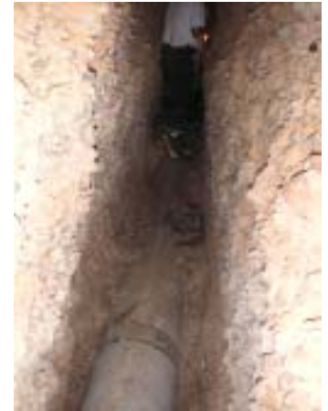
Gallery before pipe laying
