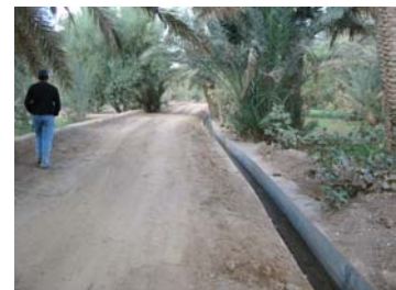
Rehabilitation of irrigation canal (Concrete canal)
