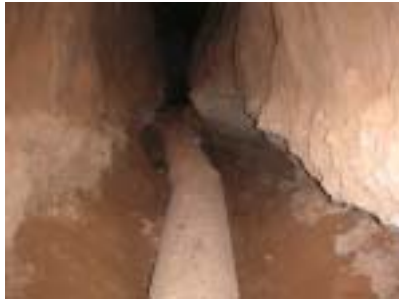
PVC pipe laying (Excavation and smoothing bottom surface before pipe laying)
