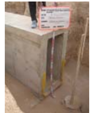
Section of gallery (Height: 1.5m, width 0.6m)
