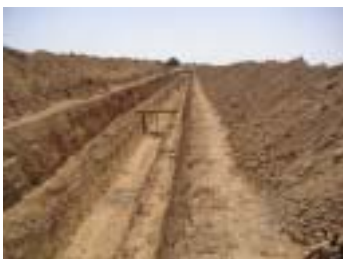
Galley before rehabilitation (Gallery wall is susceptible to collapse)
