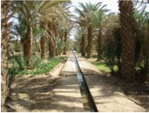
Canal rehabilitation work by concrete lining canal
