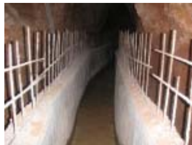
Concrete culvert for rehabilitation (Wall concrete is under construction.)
