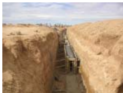
Concrete culvert construction with open excavation work
