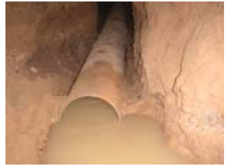
Pipe laying at 16 m deep from the ground
