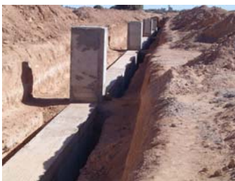
Rehabilitation of khettara (Shafts and gallery)
