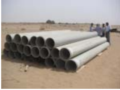
PVC pipe is available to reduce leakage loss from gallery
