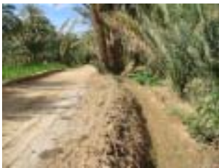
Before rehabilitation work
