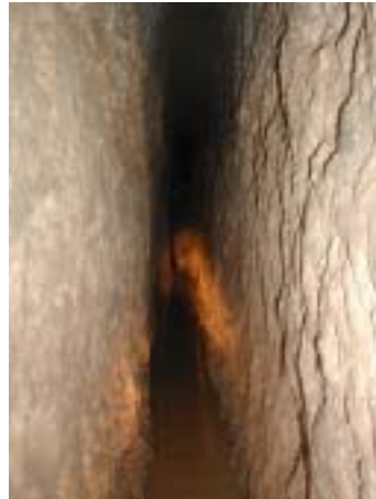
Gallery before pipe laying
