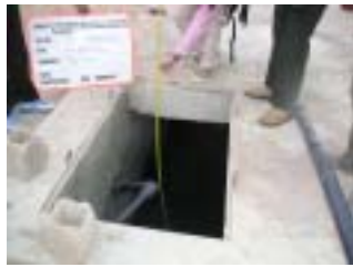
On-farm reservoir (under ground)
