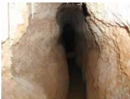
Gallery before rehabilitation works
