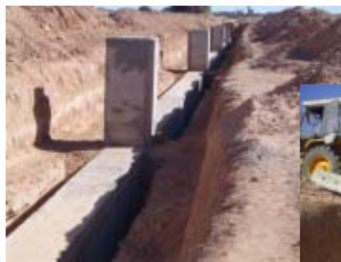
Open excavation work
