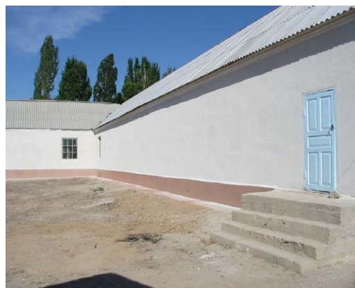
Photo 9.4 Community Center after Repair
