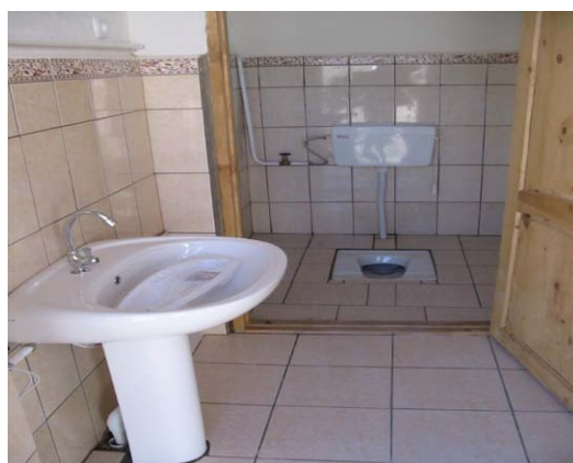
Photo 9.8 Inside the Toilet
