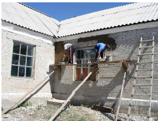
Photo 9.3 Villagers joined Repair Works
