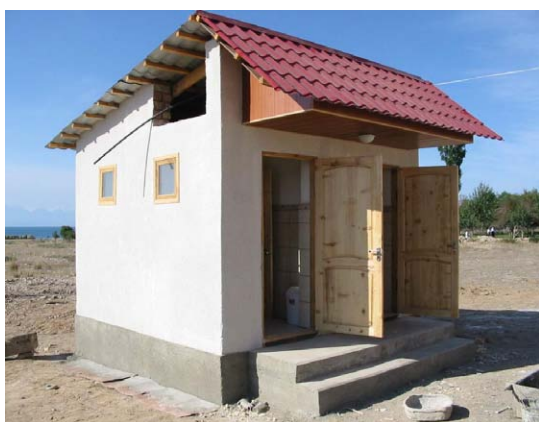
Photo 9.7 Toilet Facility beside Yulta Shop
