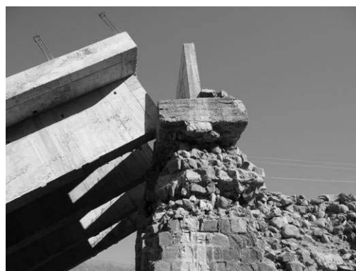
Collapsed stone masonry abutments of Subri Bridge, 6.6 km from Muzaffarabad
