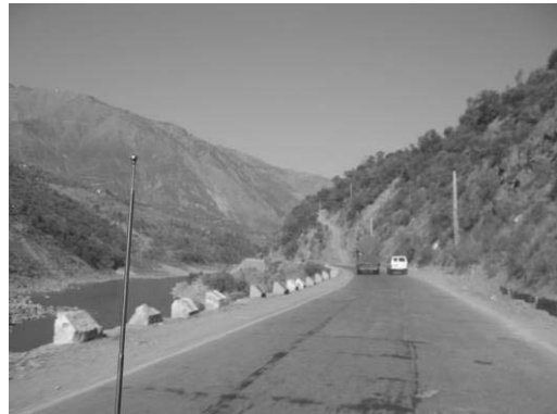
Standard section, 5 m carriageway and 1-1.5 m shoulders
