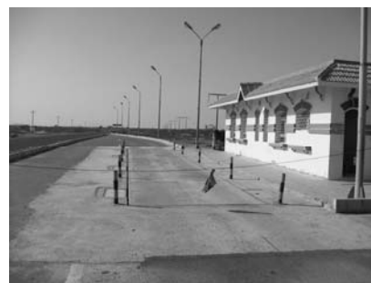
Weigh Station on the N-25
