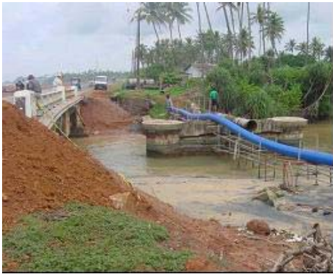
View of the Site
