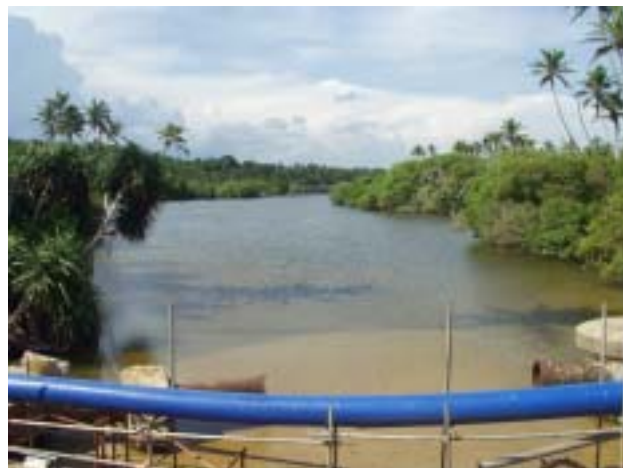
Photo-3: Left Abut of Wellamadama Bridge, view from downstream
