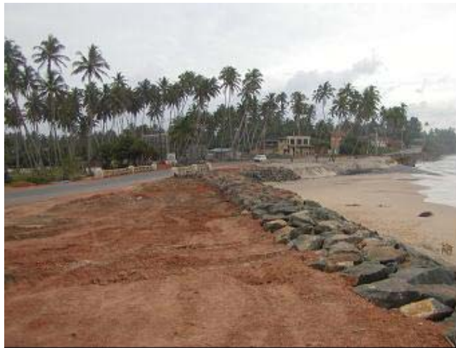
Photo-8: Wellamadama Bridge (National Road No.2) and Seashore
