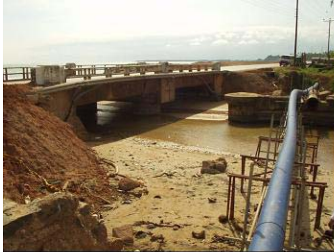
Photo-4: Wellamadama Bridge and Temporary Aqueduct, view from left bank
