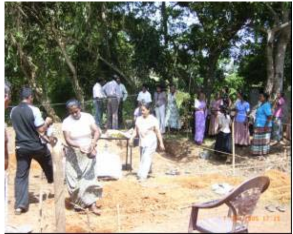
Foundation laying activities by the members
