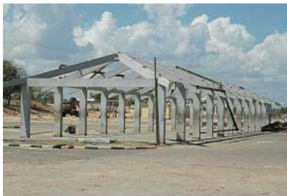
Figure 8.18 Damaged Auction Hall of the Kirinda Fishery Harbor
