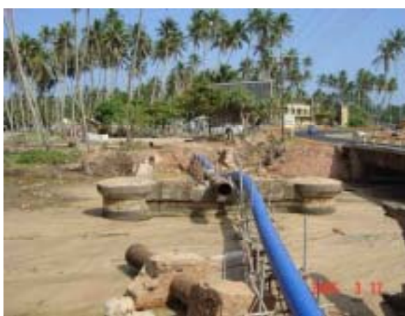
Note: The photo shows a temporary pipe and support at low tide.
