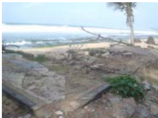
Figure 10 Collapsed Fishery Cooperative Bank Office Building in Epitamulla
