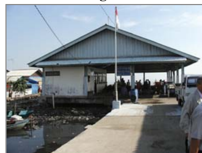
Facility of TPI Stand
