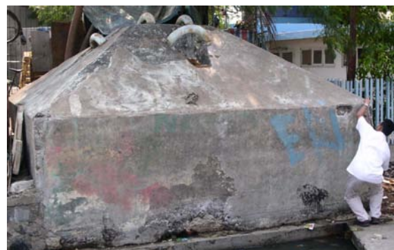
Photo 6.4.1 100t Concrete Block Sinker (10 th October 2005)
