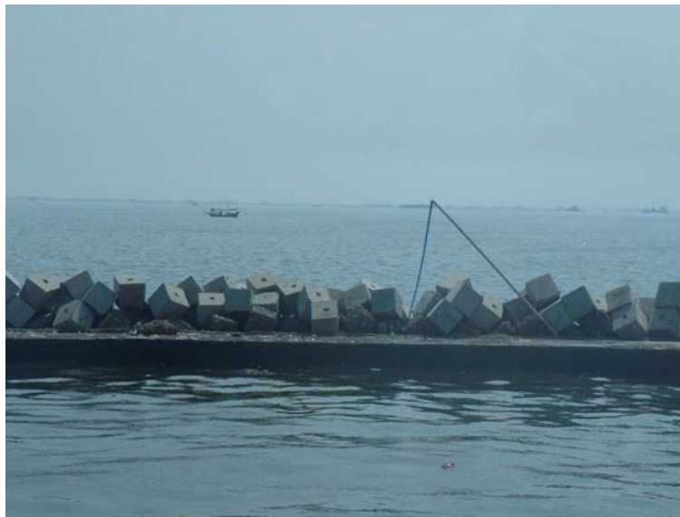
Photograph of Existing Dam Timur toward offshore side
