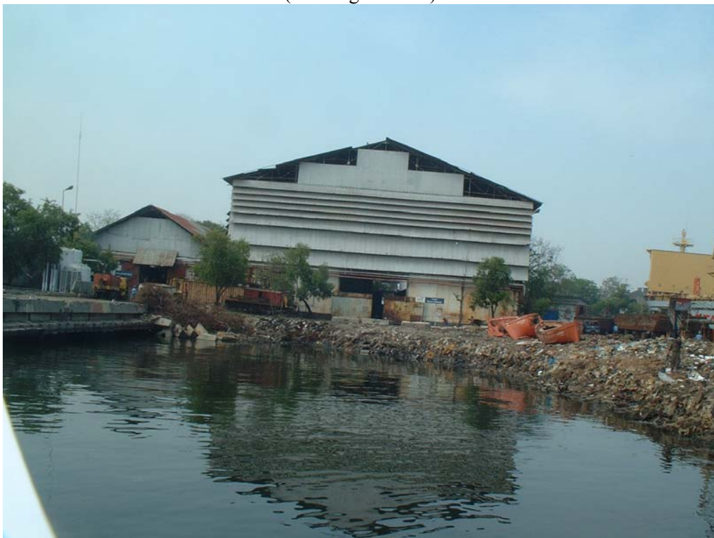
Photo 3.5.3 Possible Location for Sector Light Tower ● (Viewing landward)
