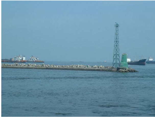
Port Entrance Marker (Dam Barat)
