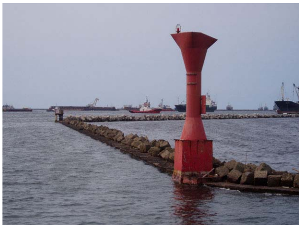
Western End of Dam Tengah
