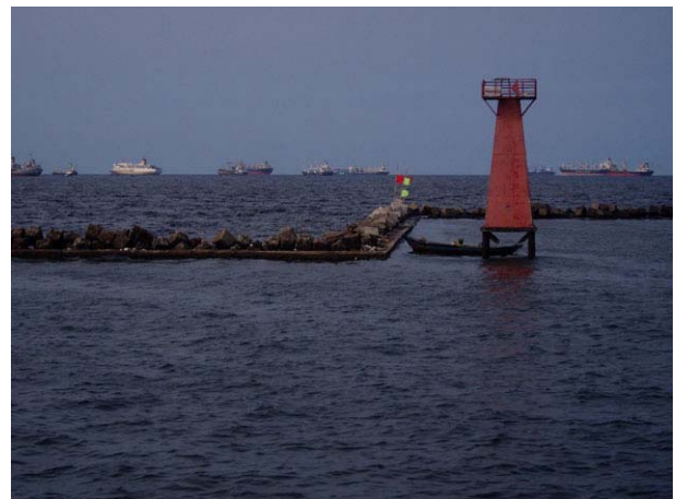
Eastern End of Dam Tengah
