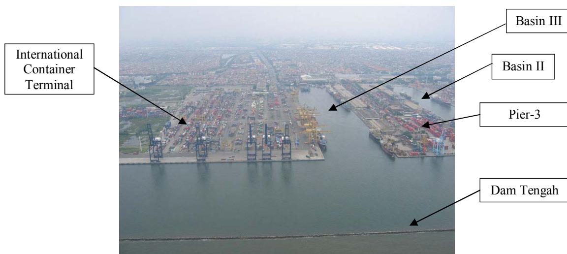
Photo 4.1.3 Existing Breakwater (Dam Tengah)
