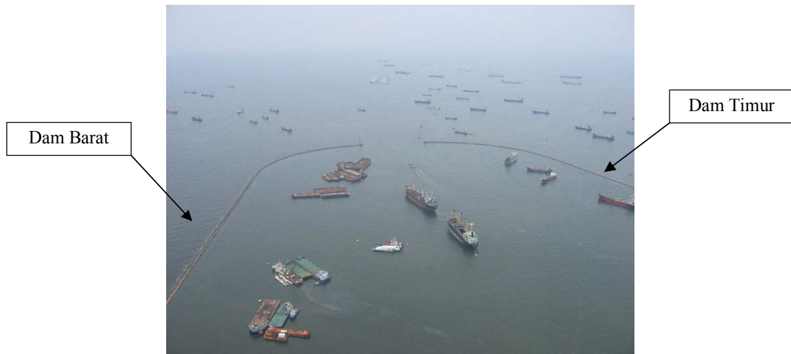
Photo 4.1.1 Existing Breakwater (Dam Barat & Dam Timur)
