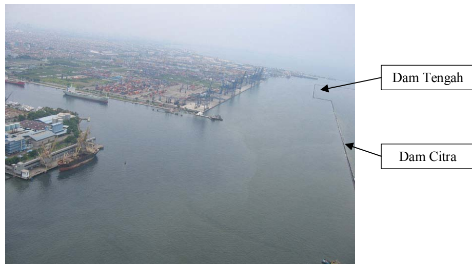
Photo 4.1.2 Existing Breakwater (Dam Tengah & Dam Citra)
