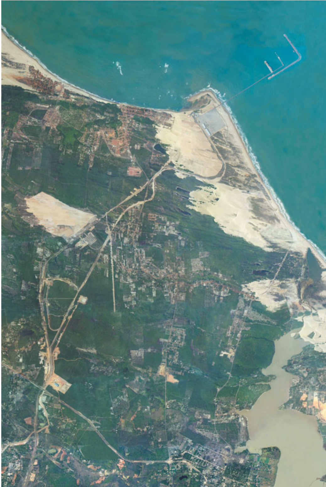
Pecem Port and its Surroundings
