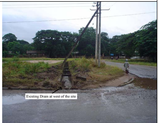
West Corner of the Front Road
