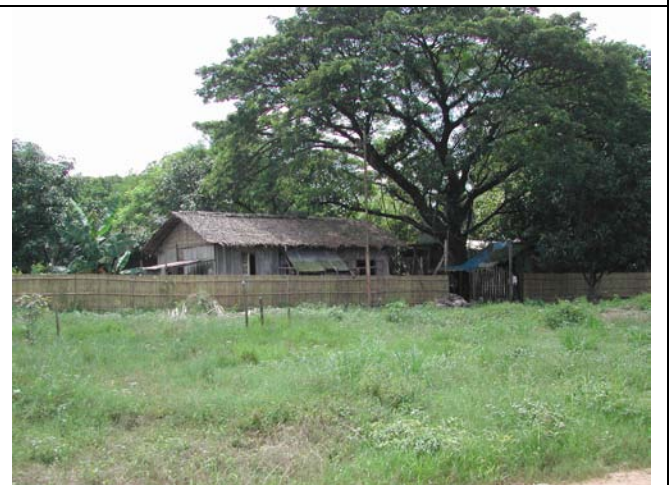
Existing Building at the South Side
