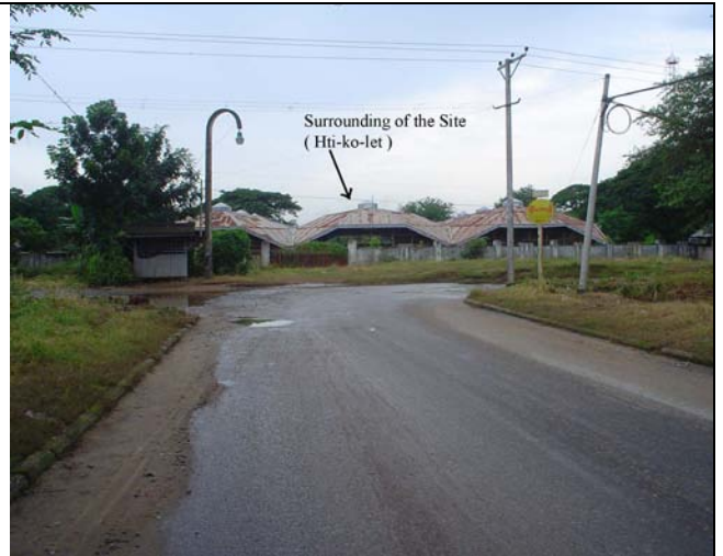
Looking West from North Front Road
