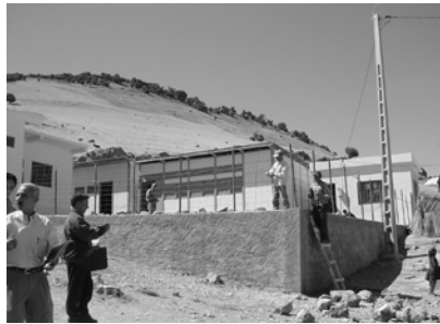
Prov. Khenifra Moulay Yacoub Construction of retaining wall and fence
