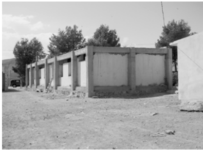
Prov. Boulmane Enjil Ikhataran Reinforcement of structure for prefabricated classroom
