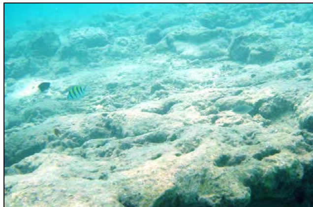
Fig. 1.5 Diving investigation for Damage Island Harbour Structures - 2
