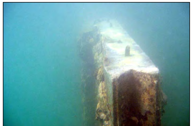
Figure 1.4 Diving Investigation of Damage Island Harbour Structures - 1
