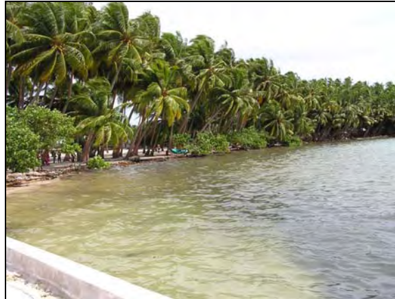
Coastal Erosion Along the Coast Adjacent to the Harbour (Photo taken in May 2005)
