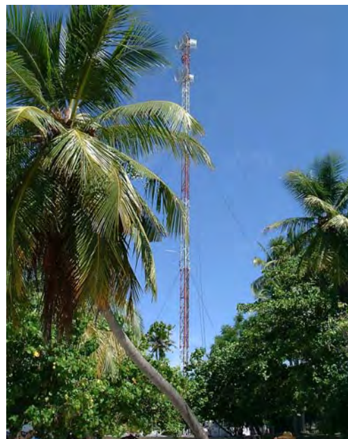
Repeater station at Felidhoo
