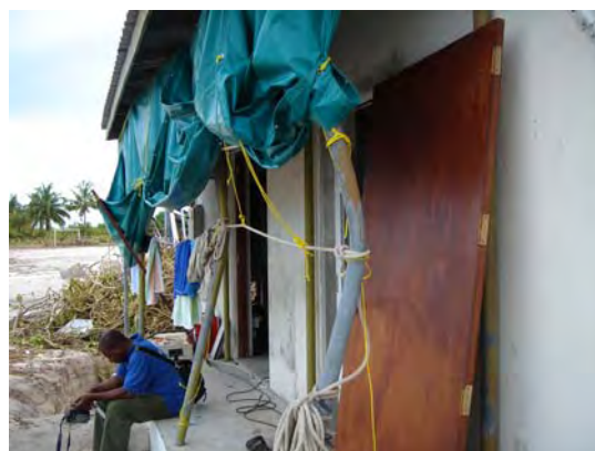
Raiymandhoo building supporting pillars
