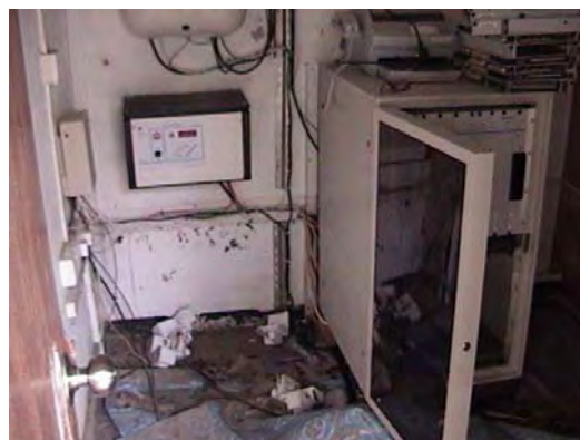
Gaafaru Equipment Room
