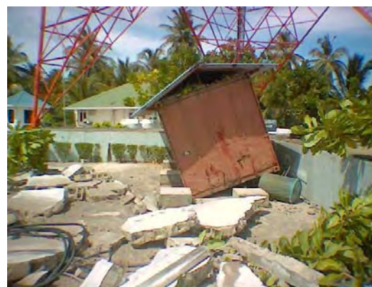
Gadhdhoo site boundary destroyed
