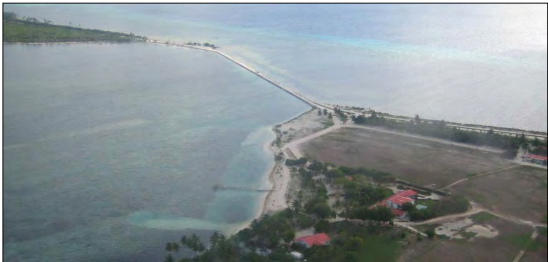
Causeway No.2 View from the north
