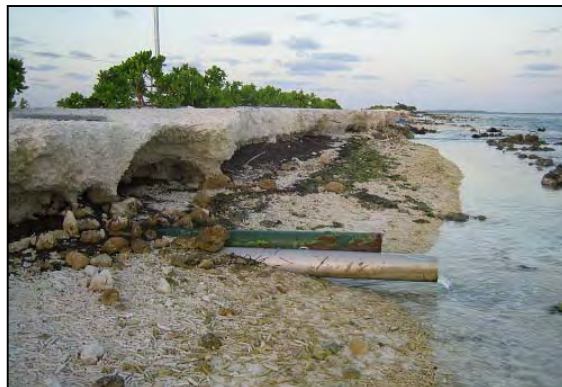
Damaged Causeway No.2 Before repair in the end of May. West side
