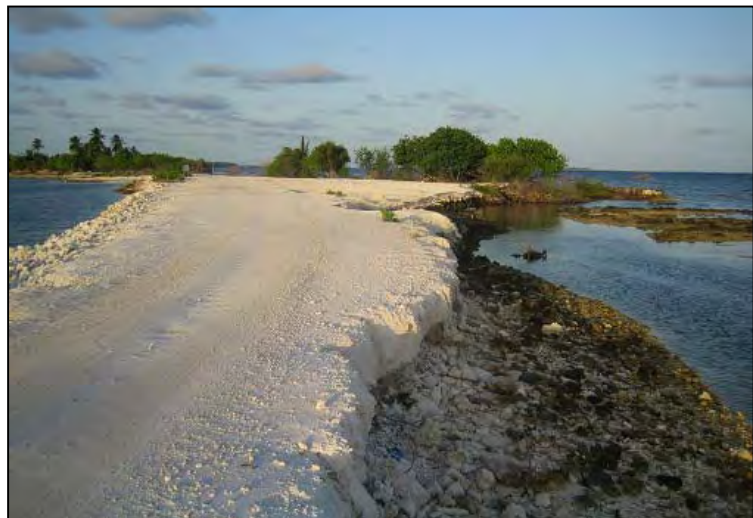
Causeway No.2 in May 20, 2005 View from the North
