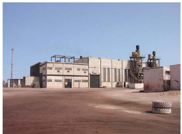
6. Nouadhibou Power Plant
