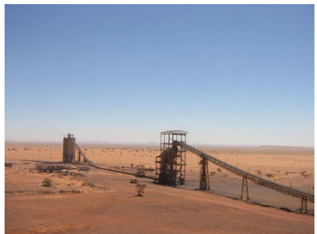
6. Secondary crusher (front) and loading hopper (behind)
