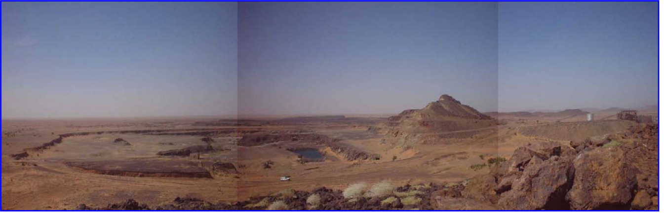
Open pit at the Akjoujt mine (Guelb Moghrein deposit). Having a small diameter of 400m S-N (left to right in the photo) and large diameter of 500m E-W, the mine was excavated until 1978. Currently, it is closed.
